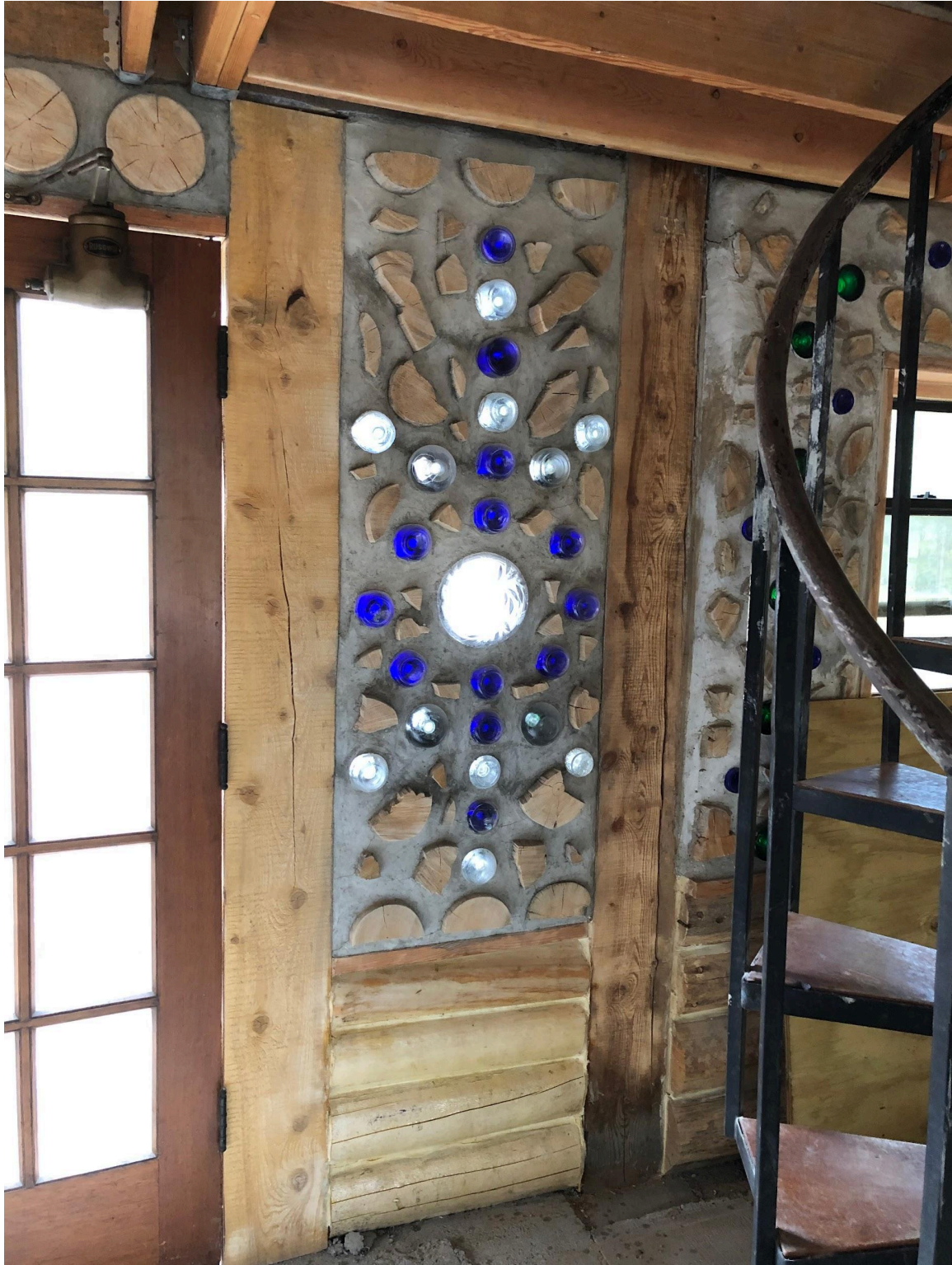
(Examples of our Cordwood Masonry using our own trees and recycled bottles)
