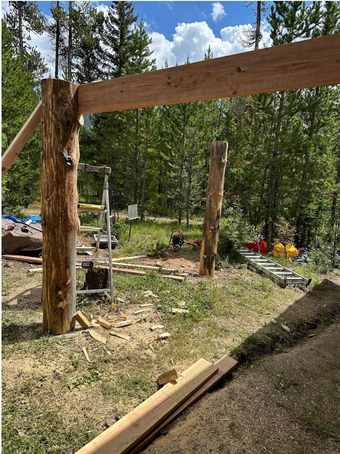
Deck began with two large tree trunks harvested from deadfall in the forest placed on poured concrete pillars.
